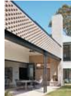
Tim Stewart Architects Mahara Street p.226
